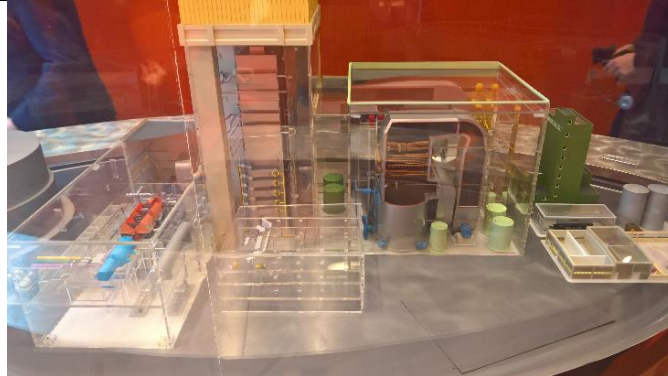
Model of biomass CHP plant
